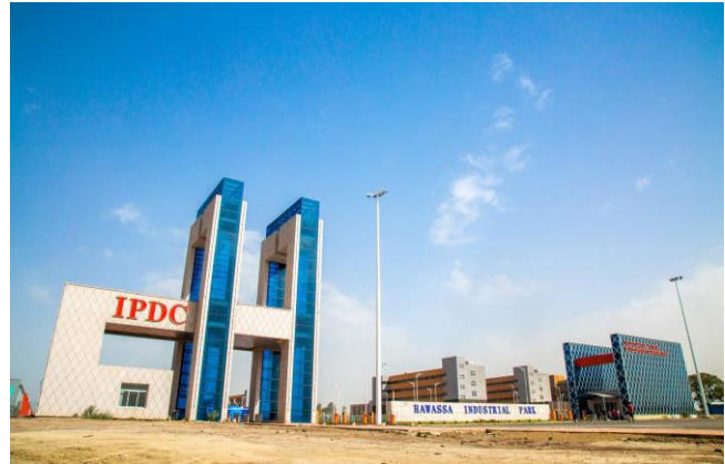
Hawassa Industrial Park
