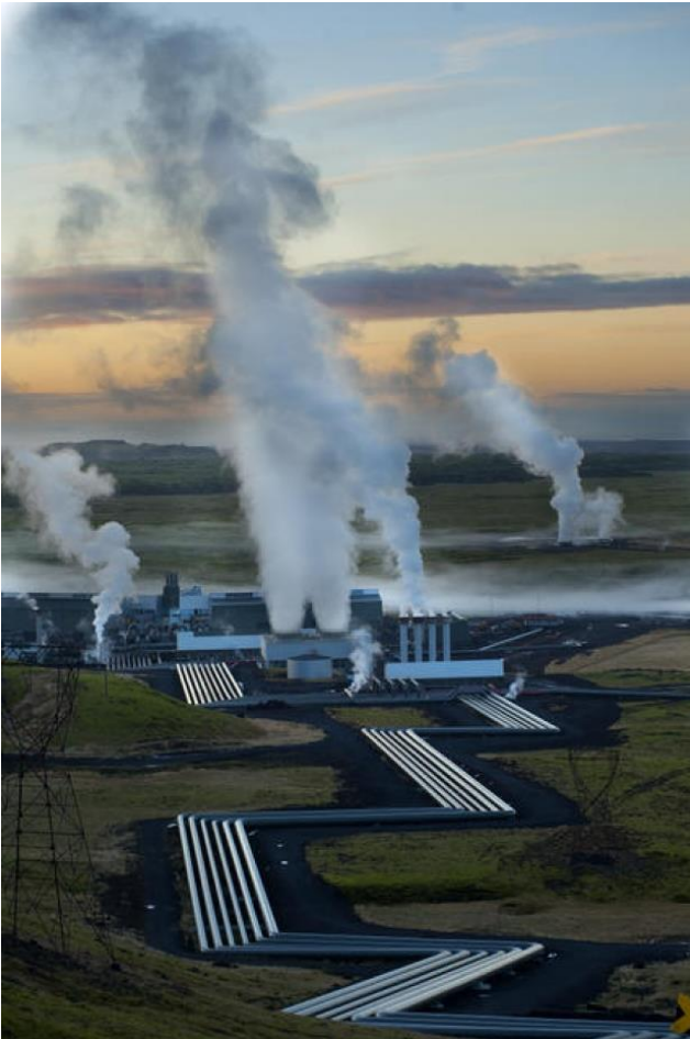
A geothermal power plant in Iceland. Photo: Páll Stefánsson.
